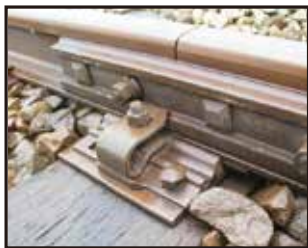
Installed with ordinary nuts
